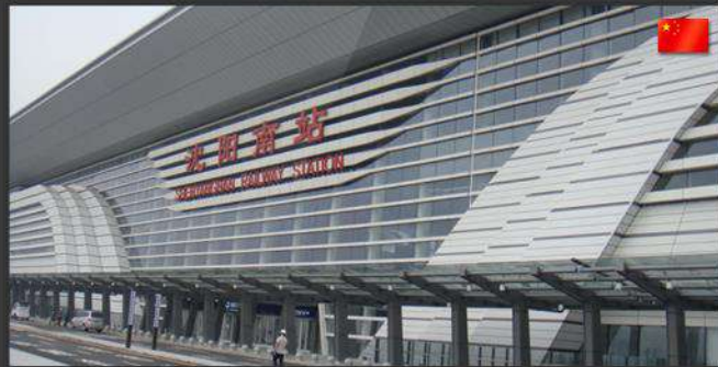
Shenyang Railway Station
