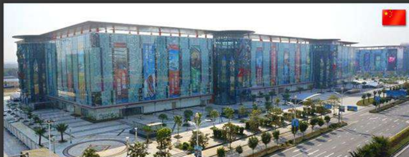
China South City Mall (NANNING, SHENZHEN, HEFEI, HARBIN) Centrifugal 287 900 кВт / 2011~2015
